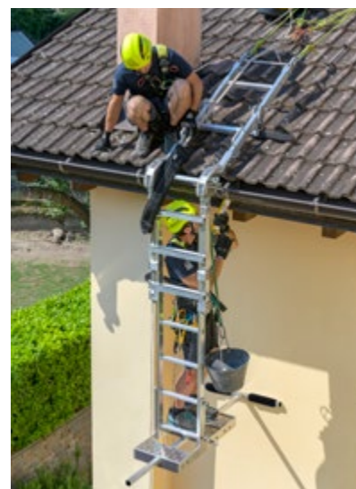
Work under the eaves.
