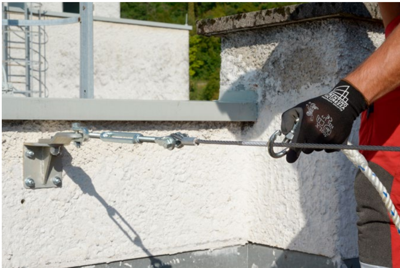
TsSafe with wall plate on a reinforced concrete structure.
