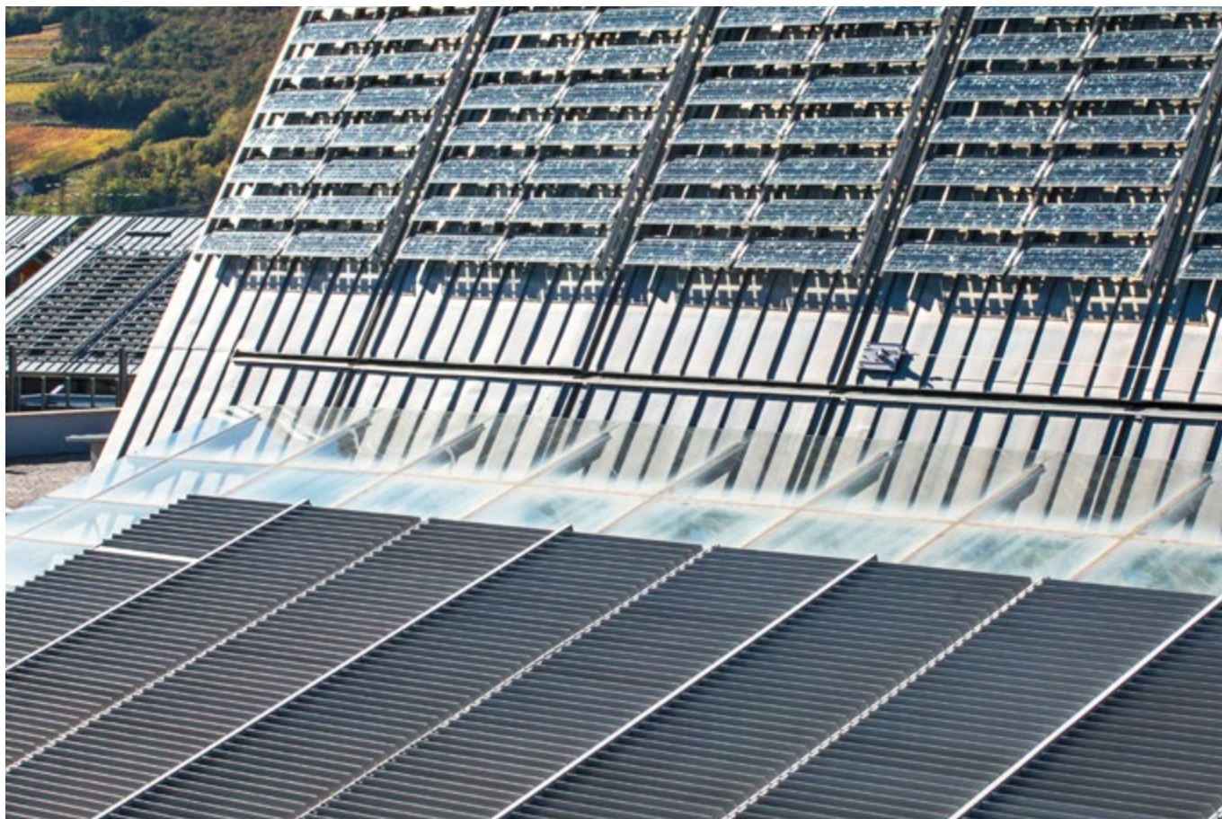
TsSafe for standing seam metal roofs Type 1 on a steep-slope roof.
