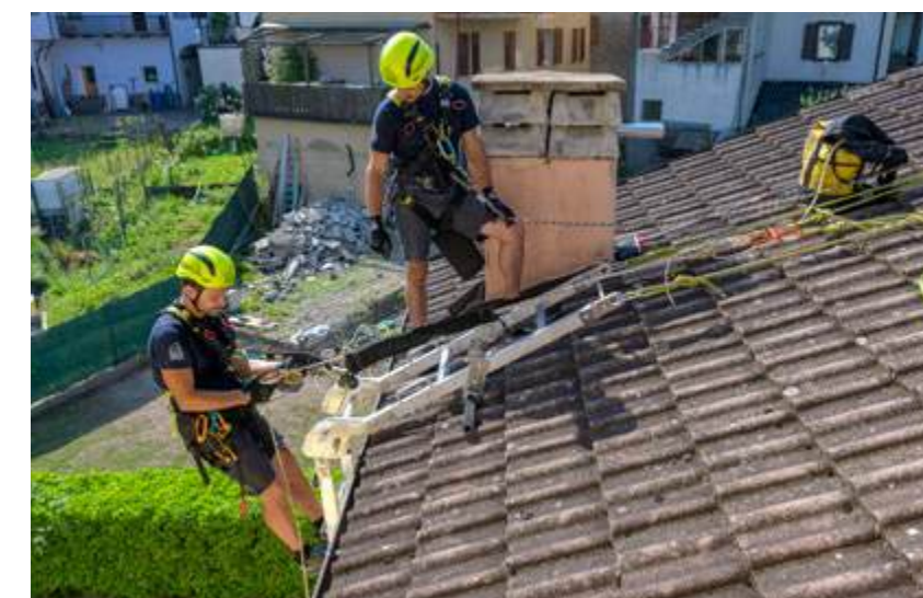
Access to the work area.
