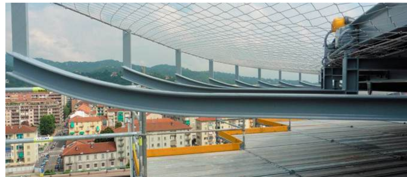
Safety net installed in cantilever configuration.
