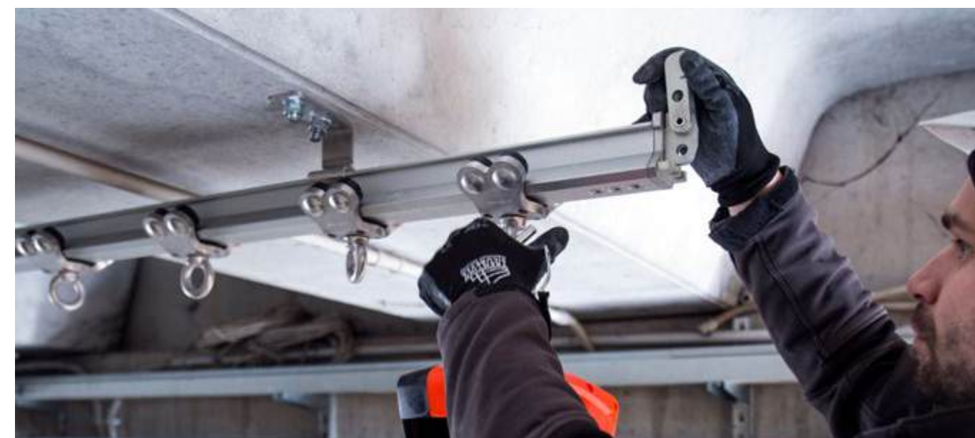
RailSafe installed on a reinforced concrete structure with Type 1 bent brackets.
