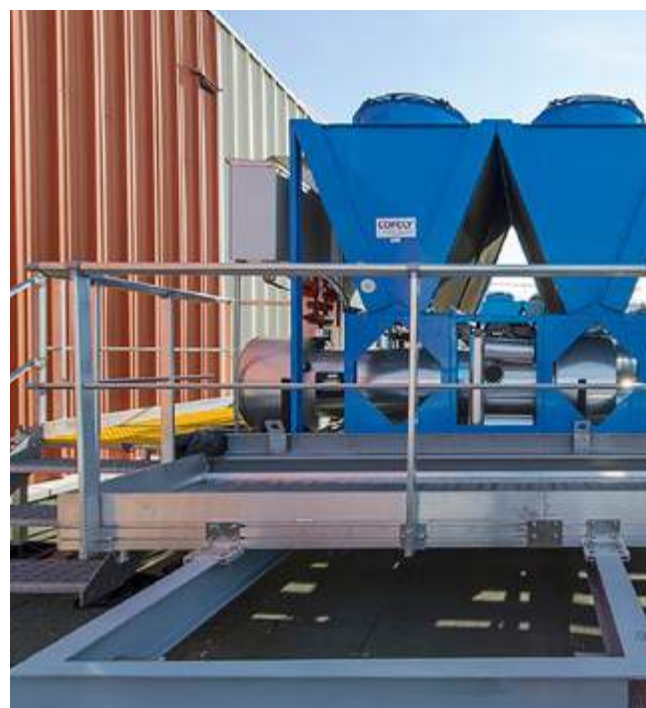
Straight guardrail, wall-mounted.
