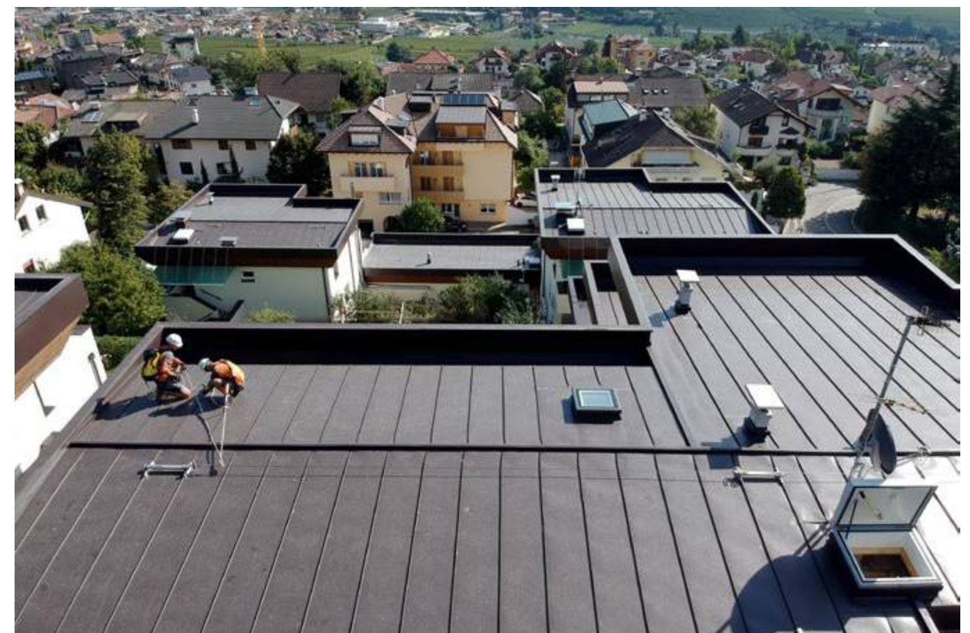
TsSafe for standing seam metal roofs Type 2 on a residential building.
