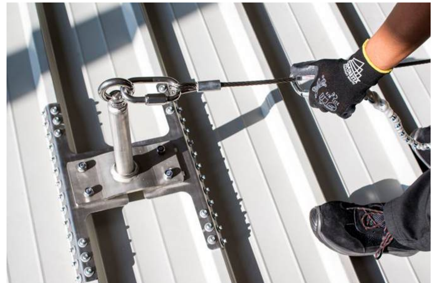
EcoSafe for corrugated sheet metal roofs on an industrial roof.
