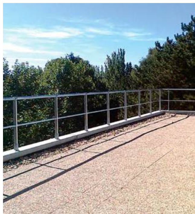
Straight guardrail, floor-mounted.
