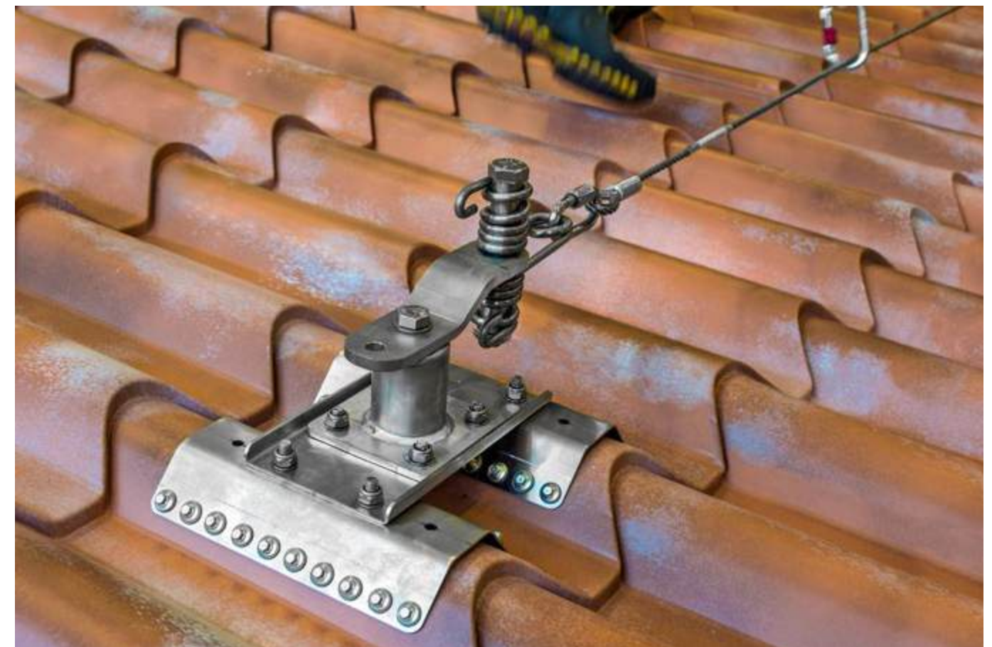
TsSafe for tile-profile sheet on a residential roof.
