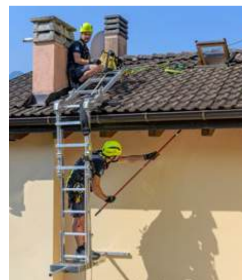
Work under the eaves.
