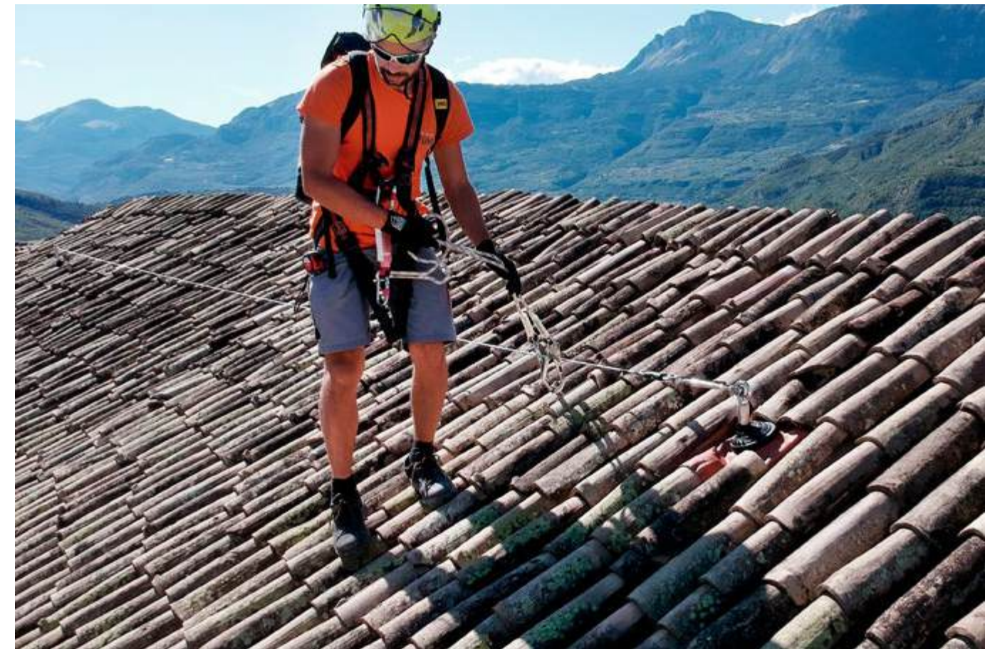
EcoSafe with ridge kit on a single-pitch tiled roof.
